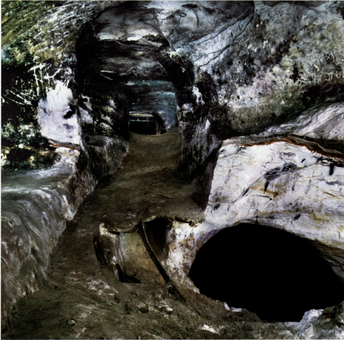
London Road mine: this view is from October 1984 before backfilling commenced. What looks like narrow-gauge railway track may in fact be support for an asphalt or cement surfaced walkway. The opening on the right leads to a lower level. Photo Nick Catford
